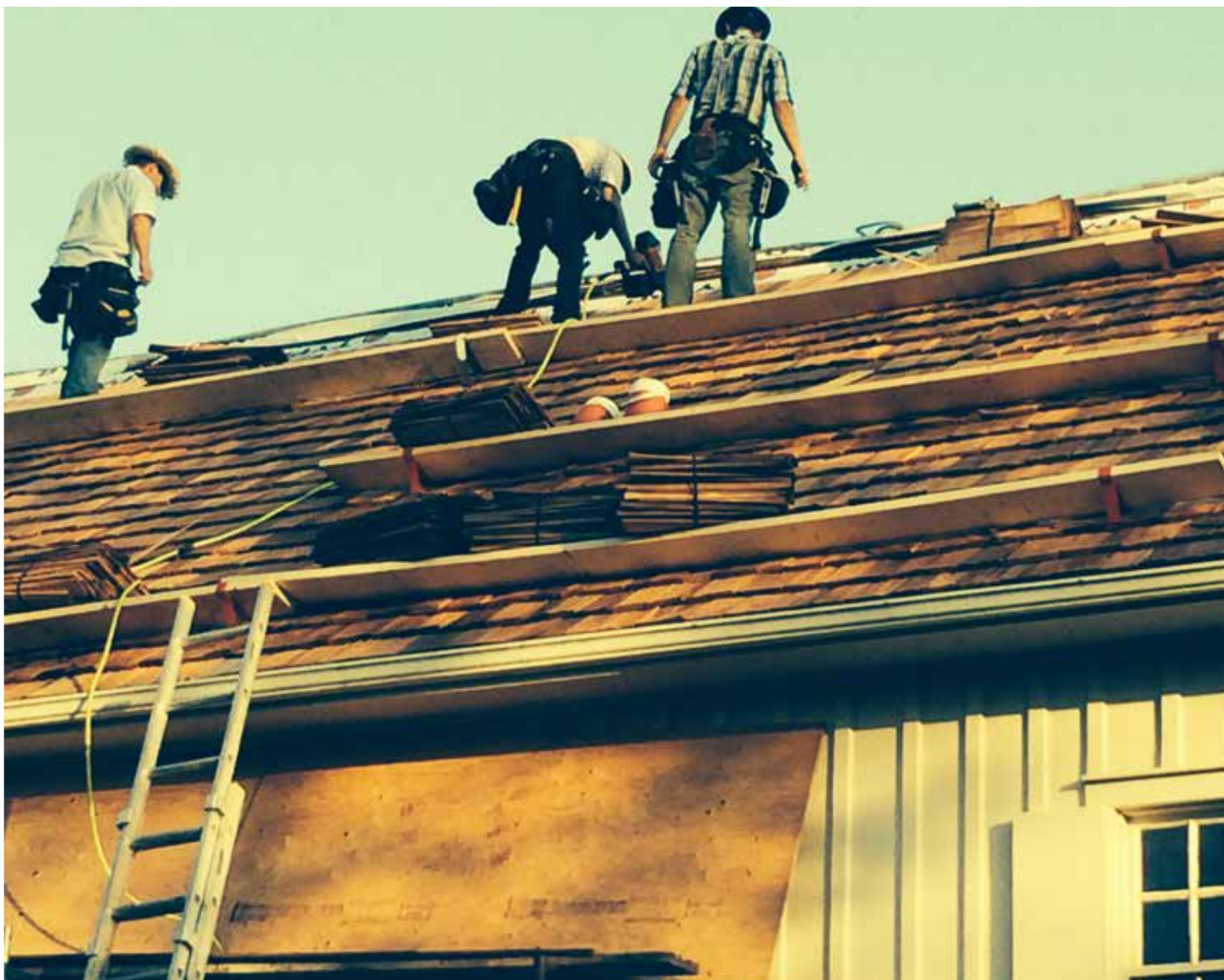
Workmen work on the 200-plus-year-old Yonge Street Meetinghouse to replace its cedar shake roof last summer.
