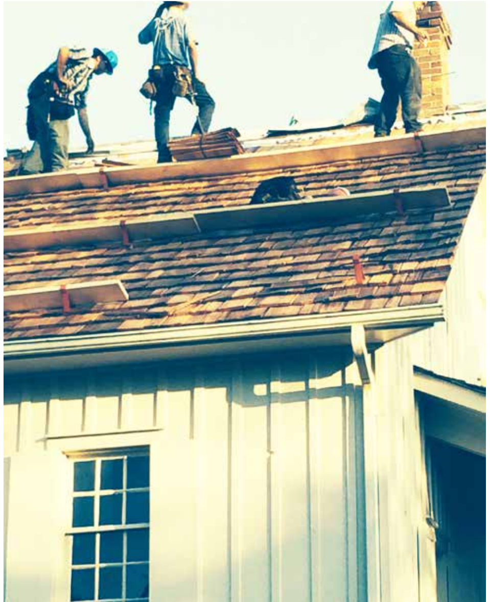
Installation of cedar shake roof on Meetinghouse completed.
